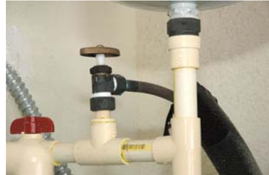
Corroded copper plumbing
