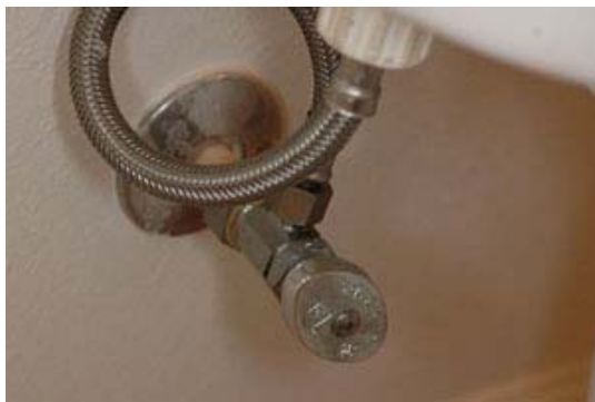
Normal shut off valve
